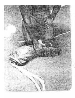
Using both hands, again form the corner at the bottom of the bag IMPORTANT: be sure to fill the bottom corners of the bag completely; this is where the bulk of the canopy should be.
